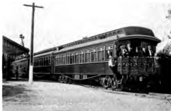
THE LIMITED AT HIGH BRIDGE. Showing the train after crossing the bridge coming north.
